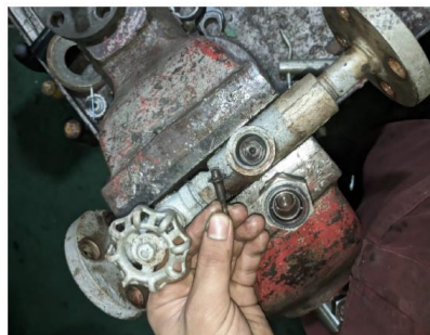
Gambar 6. Pengecekan dan perawatan steam trap
