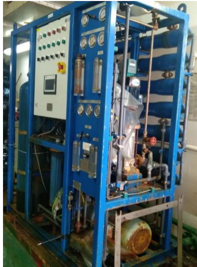
Gambar 4. Reverse osmosis plant HSRO-25E-10D
